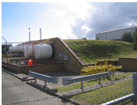
Typical Mounded LPG Tank Installation
