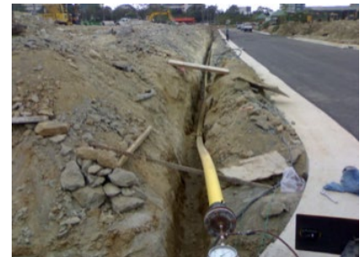
Buried PE pipe being laid
