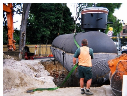
Underground LPG storage tank being lowered into position
