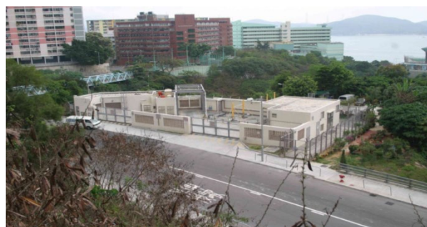
Large underground bulk LPG storage facility
