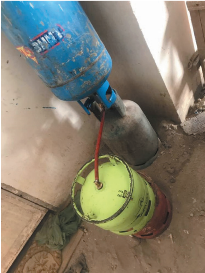
Figure 26: Illegal re-filling found taking place at Kibasila Street, Upanga area, in Dar es Salaam region
