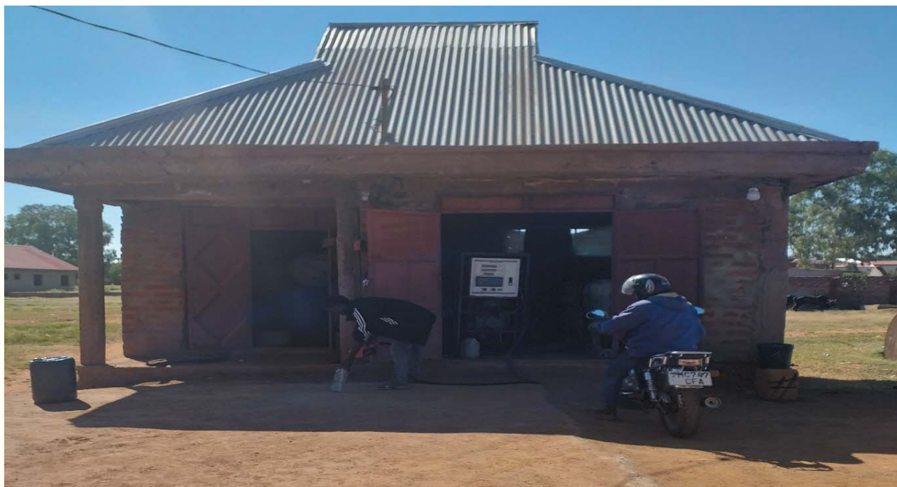
Figure 27: A residential house where plastic tanks were stored and selling of petrol was being undertaken
